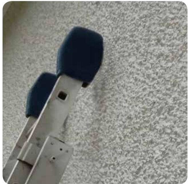
If independent scaffolds are erected using towers or similar (where access is required at height for roof, gutter, soffit & fascias replacement), protection should be provided where scaffold butts (touches) the finished scrape texture render. This will help avoid all potential damage to the finished render.
